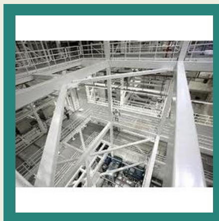
Switchyard Erection Services
